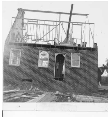
Fig 5: Rear view of masonry and framing
