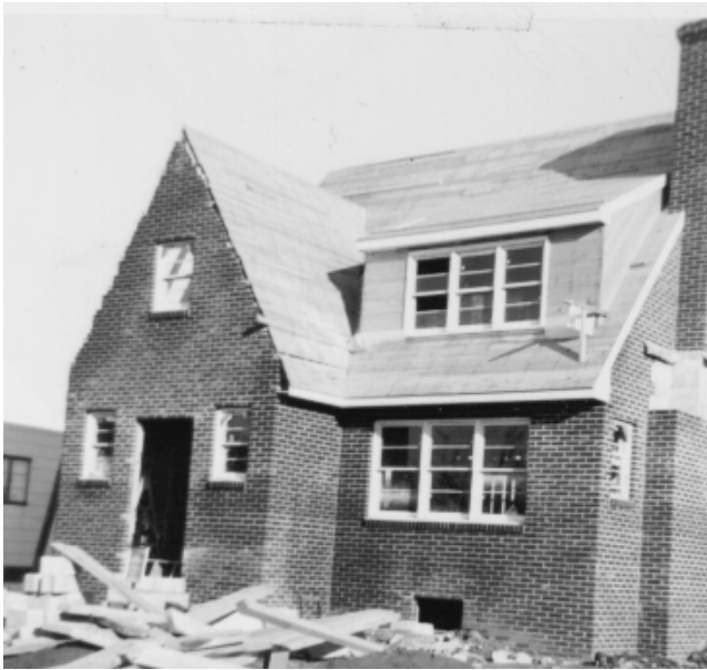
Fig. 6: View of roof sheathing
