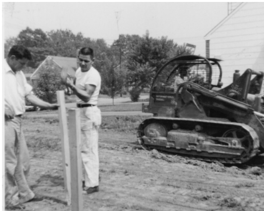
Fig 3. Start of excavation. Eddie and Pete Stevens setting
