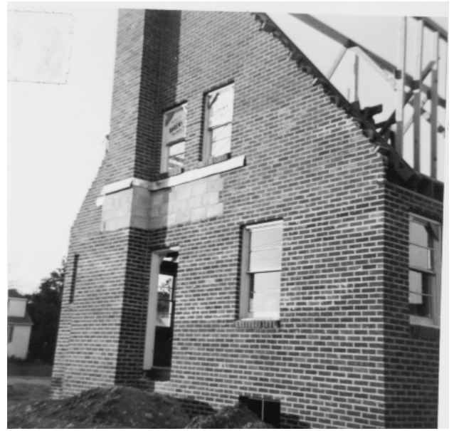
Fig 7: Rear view showing masonry and framing
