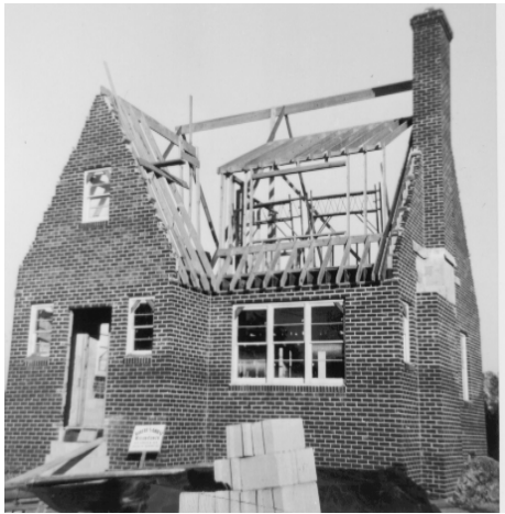
Fig 4: Front view of masonry and framing
